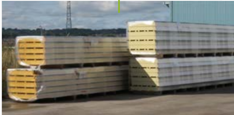
Much pre-painted metal is used for building panels and the same basic principles apply on building sites for the storage and handling of pre-painted metals. It is important to take appropriate steps to avoid corrosion and damage to panels of pre-painted metals on prior to use on the building.
